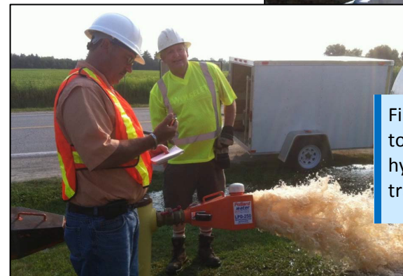
Installation of a flow meter for a District Metered Area.
