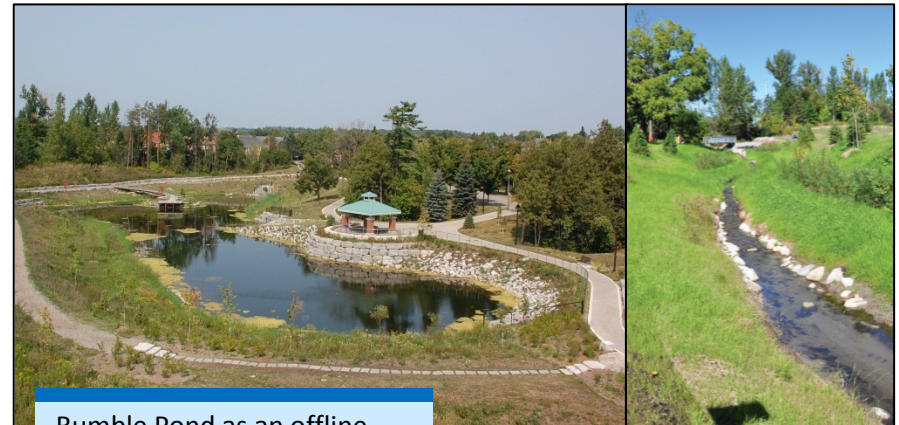
Rumble Pond as an offline facility (left); Realigned Patterson Creek (right).
