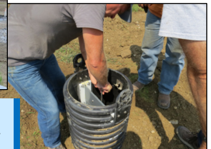
Agricultural drainage control structure for a constructed wetland.
