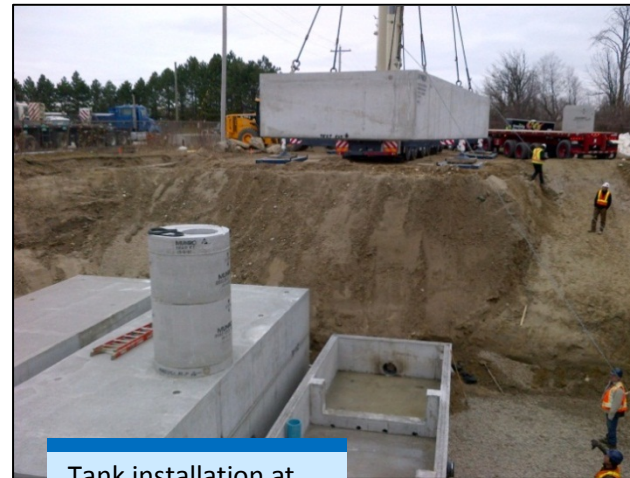
Tank installation at the Waterloo service centre site.
