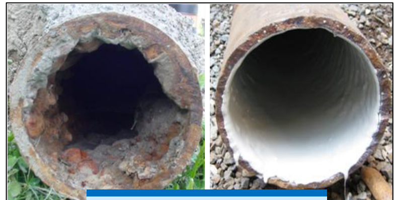
Water main before cleaning and lining (left) and Post lining (right).
